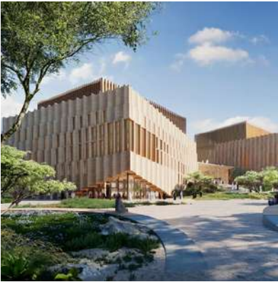
JEDDAH OPERA HOUSE (ONGOING)
